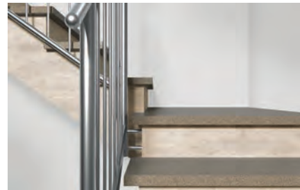
Stair treads on concrete stair stringers
