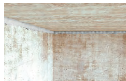
Closing joints in structural work
