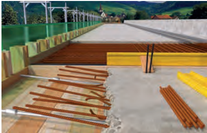
Rebar connections
