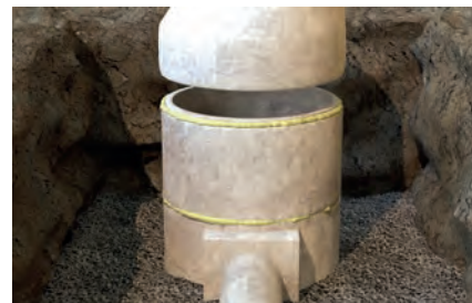
Sealing concrete manhole rings
