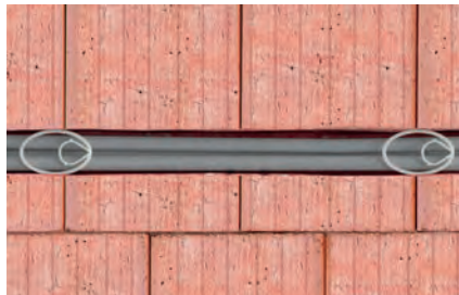
Cable fixing in wall slots > 30 mm
