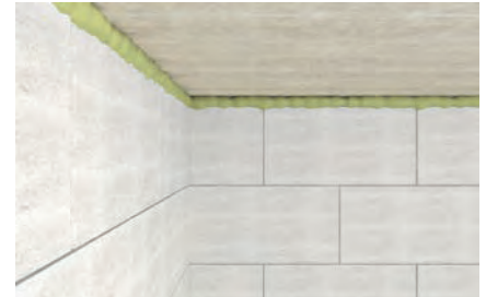
Closing joints in structural work
