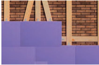
Pressure-resistant insulation boards on timber constructions
