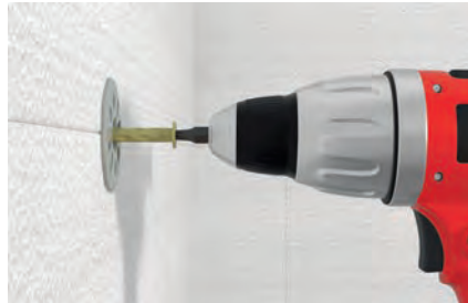
Screwed fixing of insulation boards
