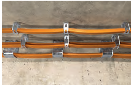
Cable fixing to the ceiling
