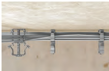
Fixing cable bundles
