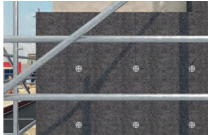
Pressure-resistant insulation boards with rendering
