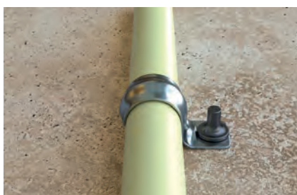
Fixing armoured conduits
