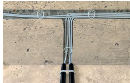
Cable fixing in wall slots < 55 mm
