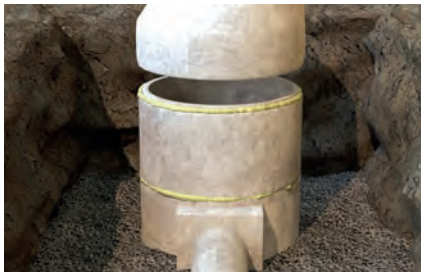
Sealing concrete manhole rings
