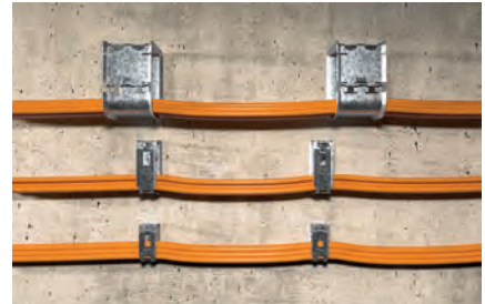
Cable fixing to the wall
