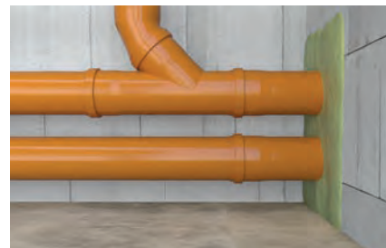
Filling pipe penetrations
