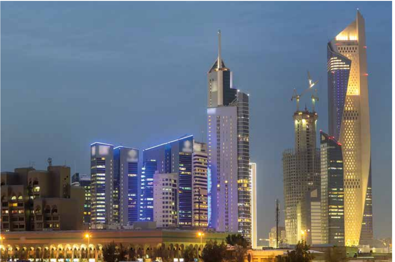
Al Hamra Tower · Kuwait
